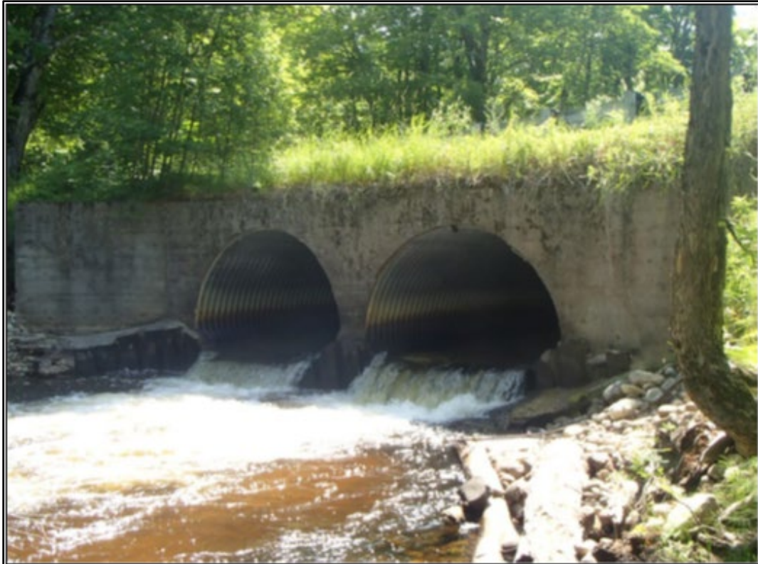
Figure 1-2. Undersized Culverts at H-58 Sucker River Crossing Prior to Replacement
