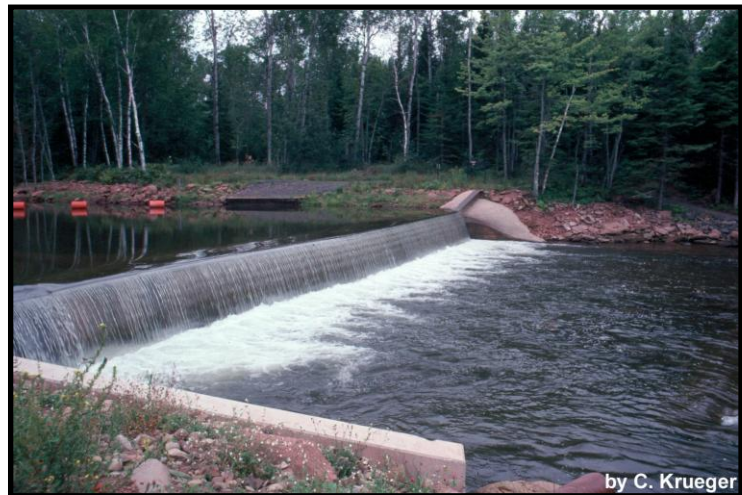
Low head barriers prevent sea lampreys from reaching their spawning grounds, while allowing fish to pass. A component of the integrated program, they help control sea lampreys without the use of lampricides.
