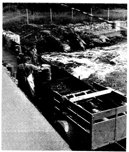
Fig. 13. Introduction of undiluted lampricide TFM from a storage tank with a constant feed chemical proportioning pump to the Kaministikwia River (near Kakabeka Falls), Ontario.
