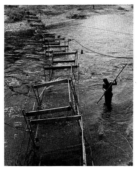
Fig. 5. Electric barrier on the Garden River of North Channel, Lake Huron. This horizontal rack-type installation, consisting of pipe electrodes and wooden separators, is typical of barriers used in Canadian waters of Lake Superior.
