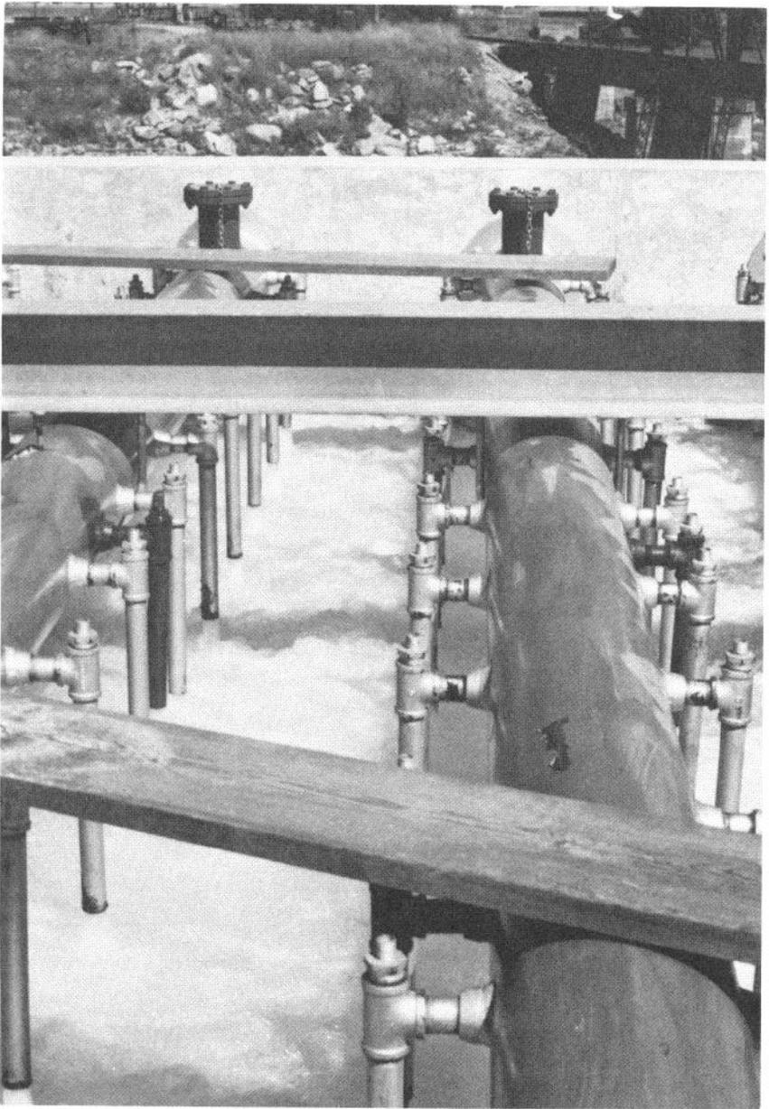
Aeration system for increasing oxygen and reducing nitrogen saturation in a hatchery water supply
