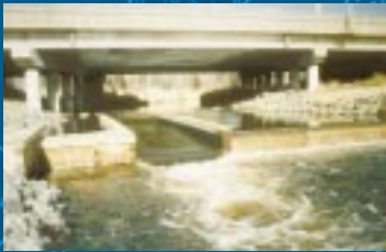
Velocity barriers exploit lampreys' poor swimming ability.
